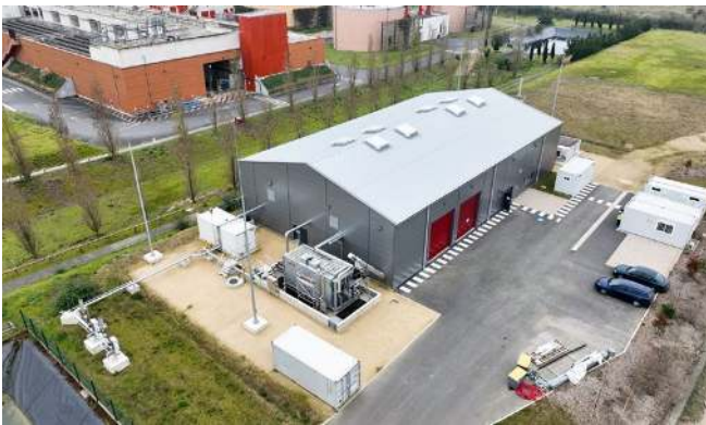
The Cométha pilot plant at Triel-sur-Seine near Paris
